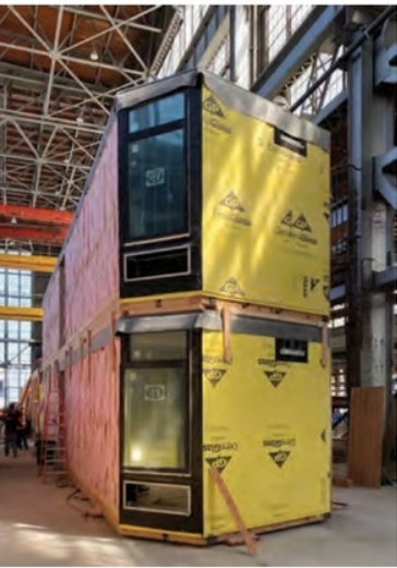
Five floors of efficient factory-built residential space are set above a first-floor commercial space built using traditional concrete construction methods.
